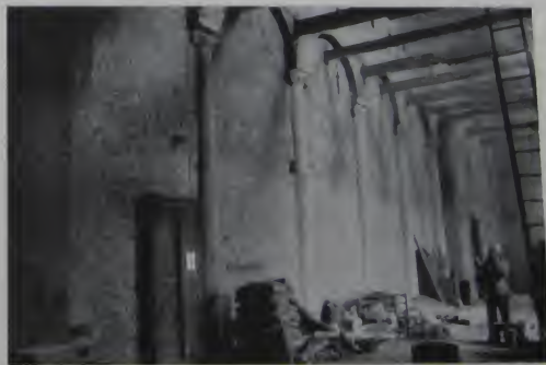
FIG. 12. EXTERIOR WALL OF THE CHOIR. NORTH-EAST CORNER.
